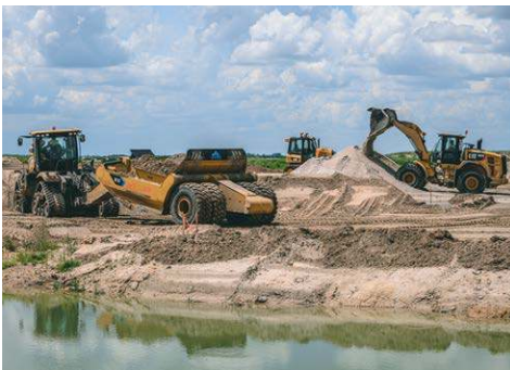
Lane was responsible for construction of the C-43 West Basin Storage Reservoir project, an Everglades restoration effort.
