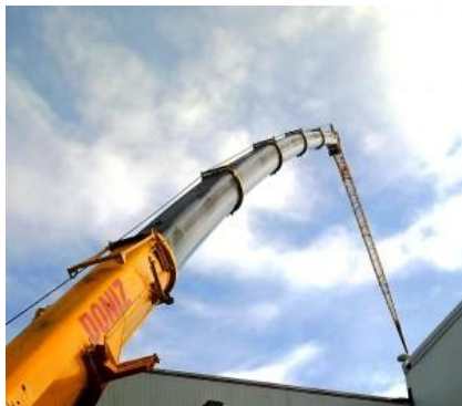
Figure 4 Example crane bending (Source: www.Craneblogger.com)
